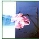
A shaker handle is used to clean the heat exchanger tubes. This is easy to do and is normally done when the hopper is filled.
